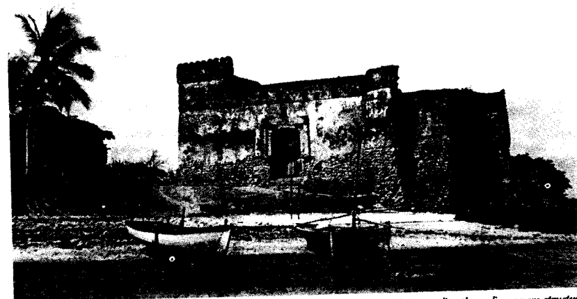
Fig. 25. The Gereza, built about 1800. Note the collapse of the round tower (right), revealing the earlier square structure of the Portuguese fort of 1505.
